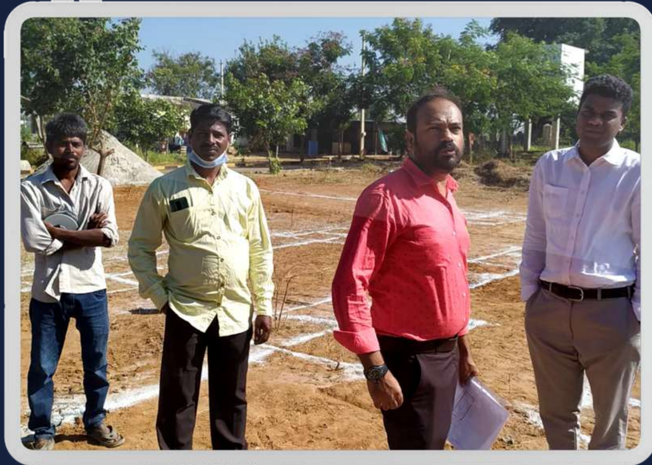
Marking for excavation of Foundation
