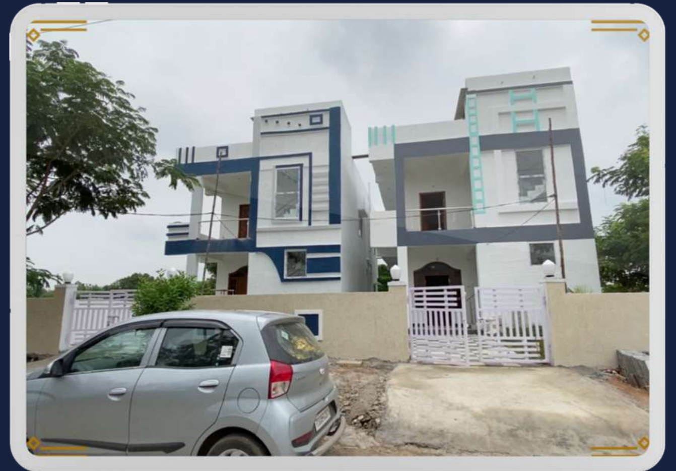
Two villas after completion
