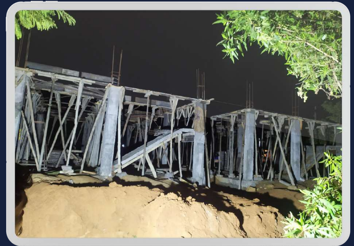
First slab work
